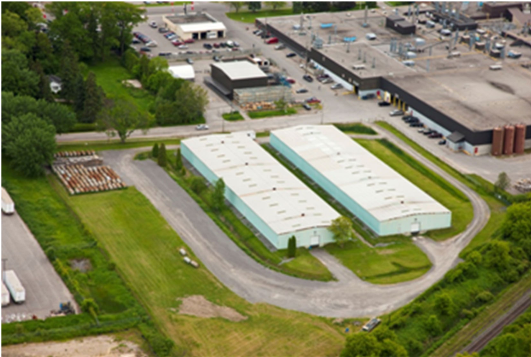
Figure 2 – Site 2 - Storage Facility
