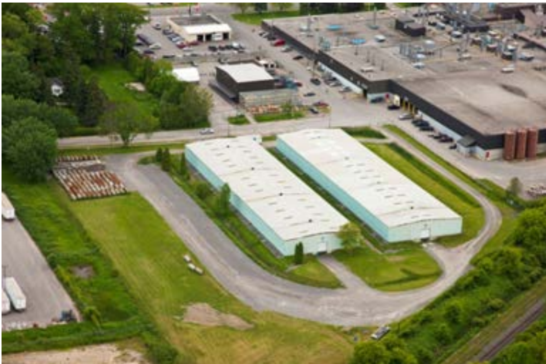
Figure 2 – Site 2, Storage Facility
