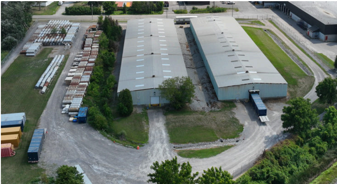
Figure 2 – Site 2 - Storage Facility
