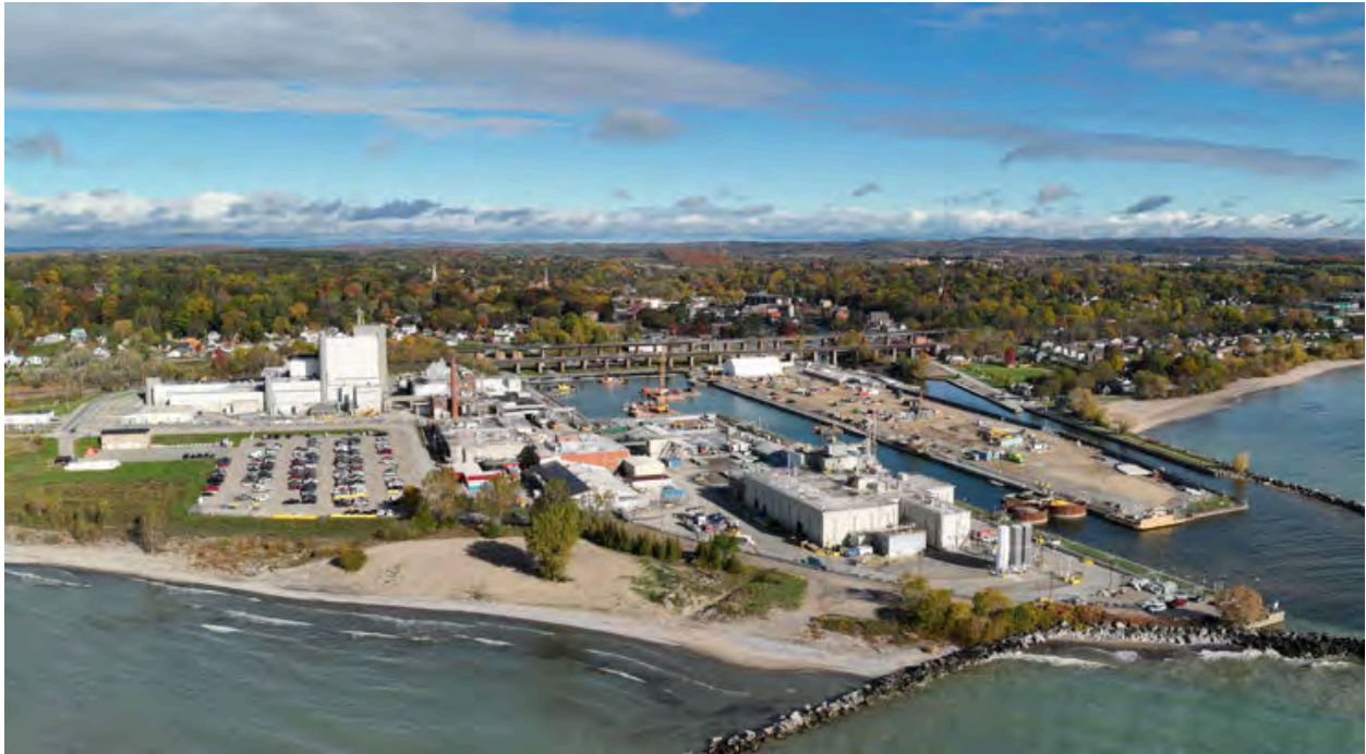
Figure 1 – Site 1 - Port Hope Conversion Facility
