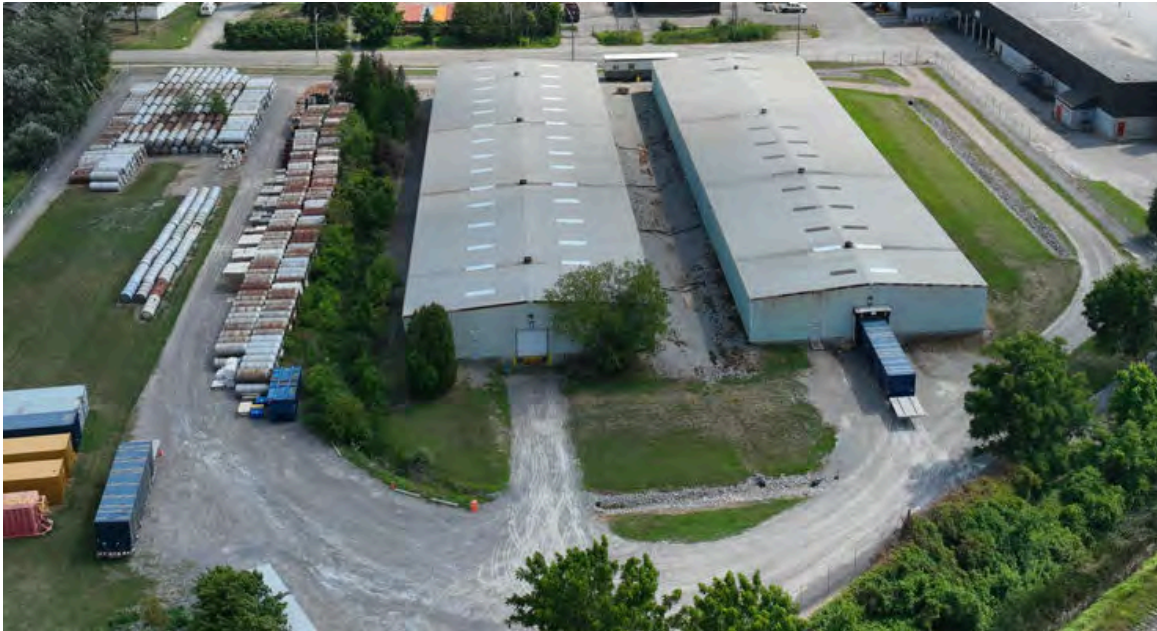
Figure 2 – Site 2 - Storage Facility
