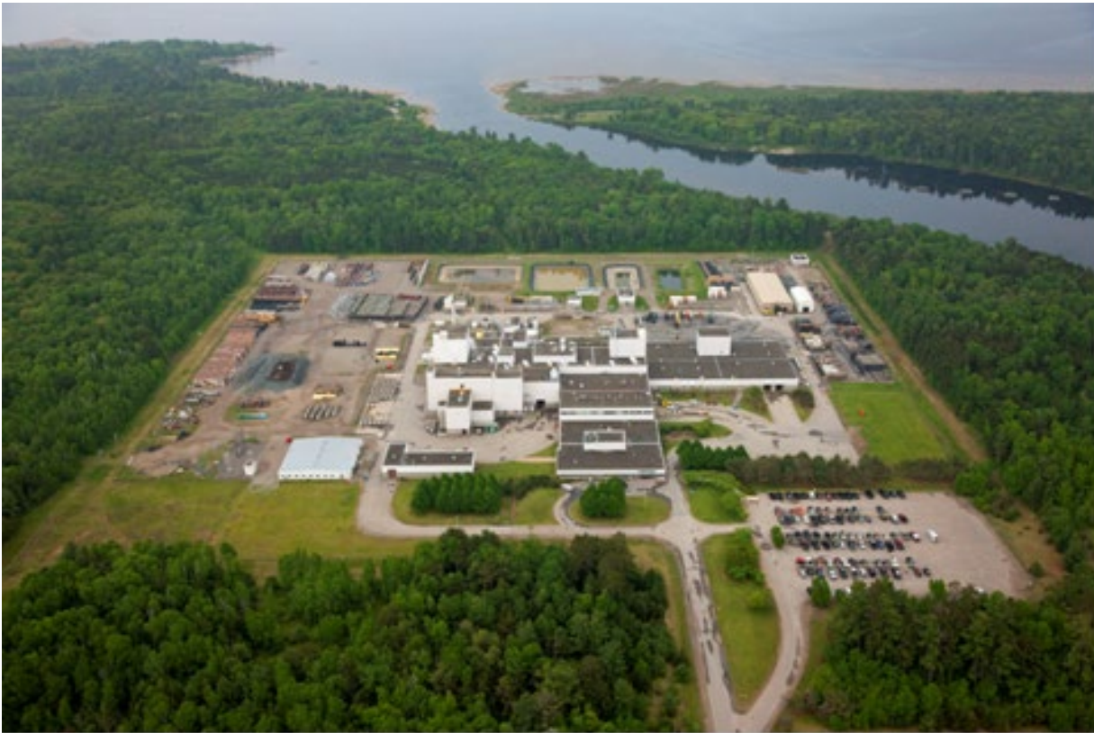
Figure 1 Blind River Refinery
